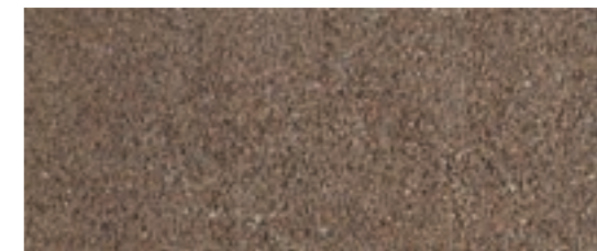
Bracken - Shot Blasted
