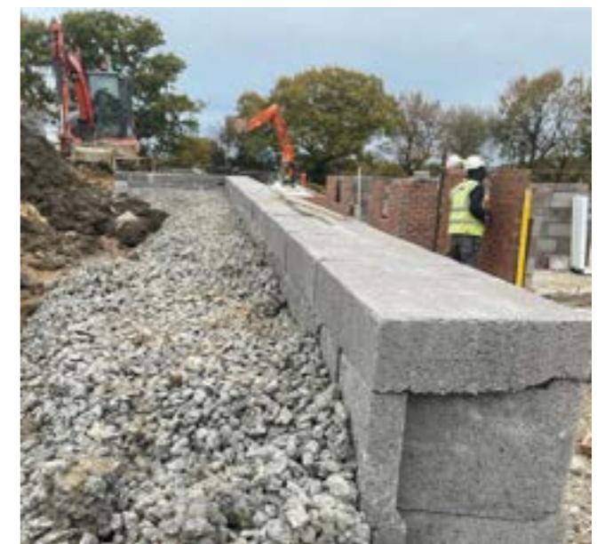
Illustrated: No-Fines Concrete installation on site
