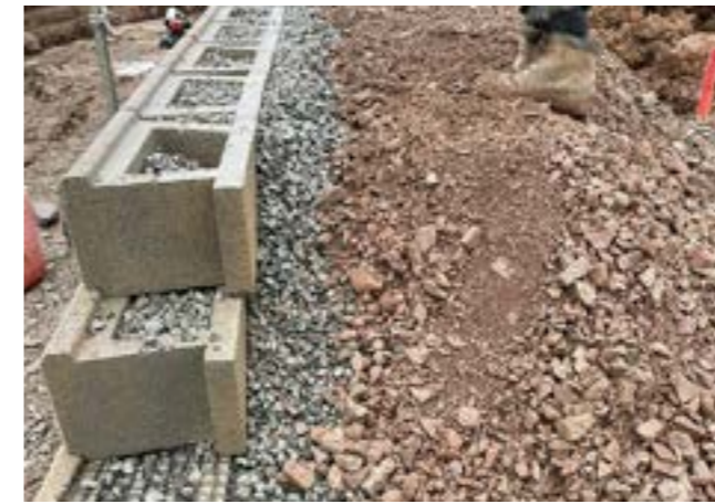
Illustrated: Geogrid Installation with backfill
