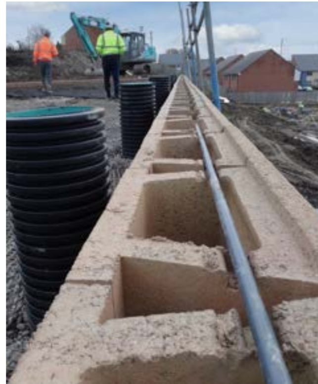
Positive Connection in use during the installation of Allan Block®
