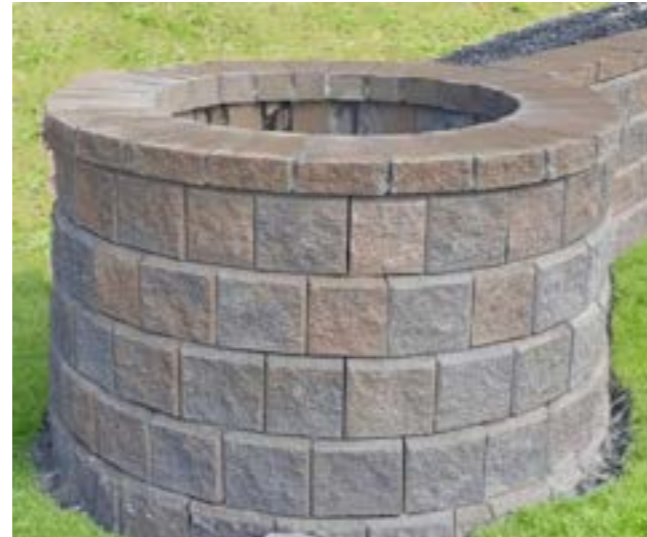
Base Course Radius for an outside curve on a 1.2m tall 6° wall
